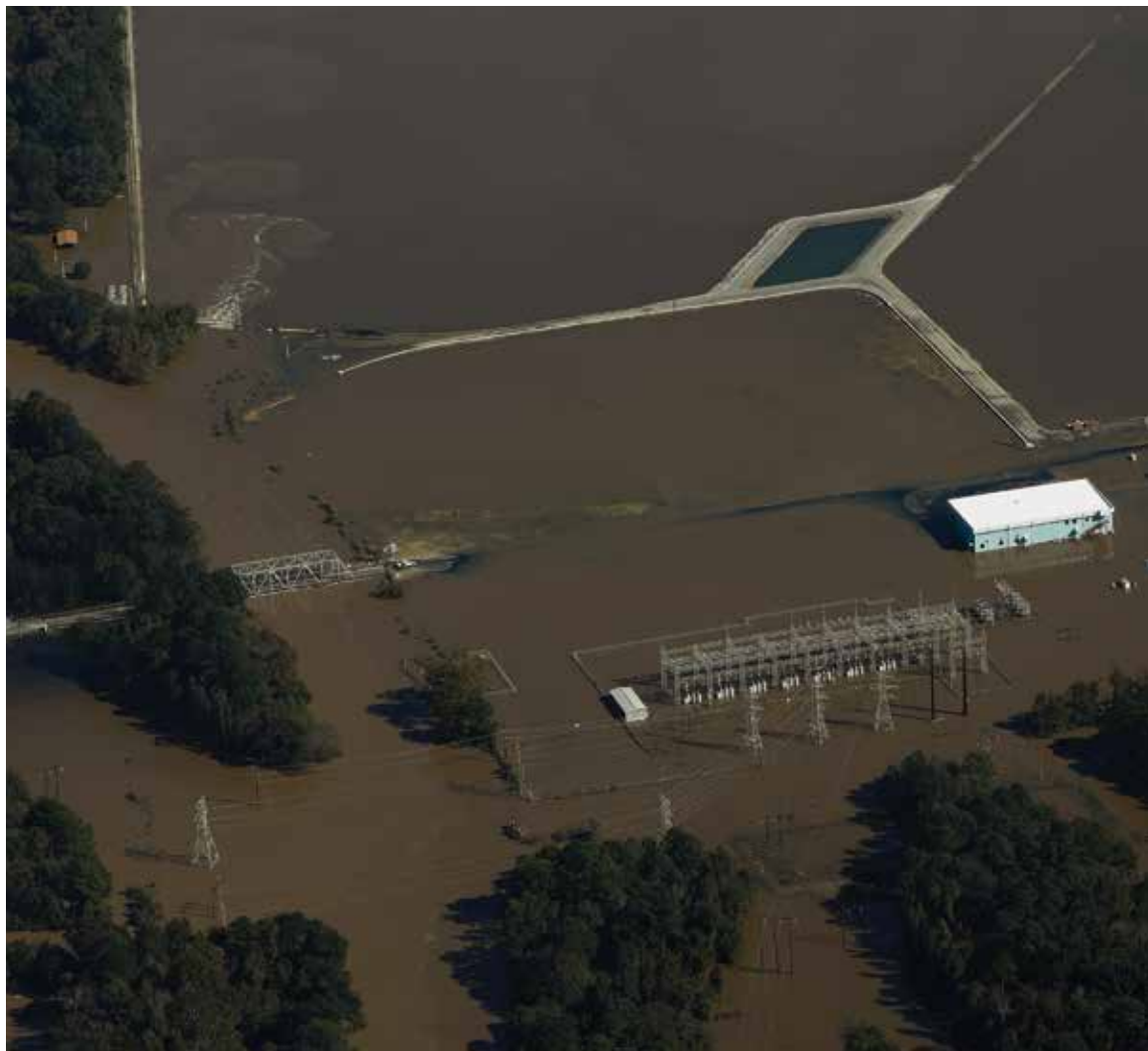
An aerial view of Duke Energy's H.F. Lee facility.
