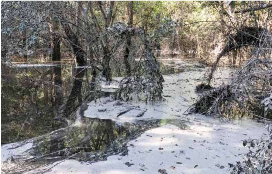
Duke Energy failed to identify a school bus-sized breach in a cooling pond dam at their H.F. Lee facility for as much as 24 hours before a local news helicopter spotted the collapsed dam and reported it to officials.
